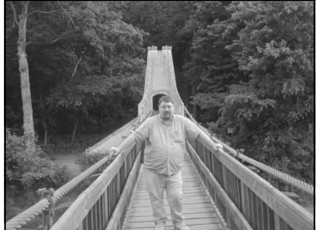
Mike D tests the Suspension Bridge for structural integrity on Friday night.
